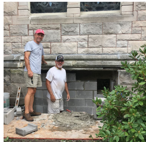
Bill Hoff and the stone mason who fixed the sagging North side of the church. It was finished off with Indiana limestone from the same quarry as the original stone and cut by Mr. Benson himself.
