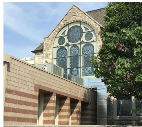
The Sanctuary has new a HVAC! We are already feeling the consistent effects.
