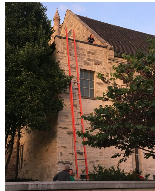
Many thanks to Bill Hoff who scaled the building to save a cat and then fixed the damage to roof he saw while he was up there.
