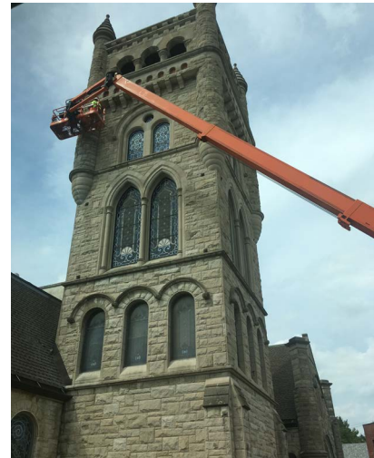
The Foundation is having work done to fix the stone falling off the tower.
